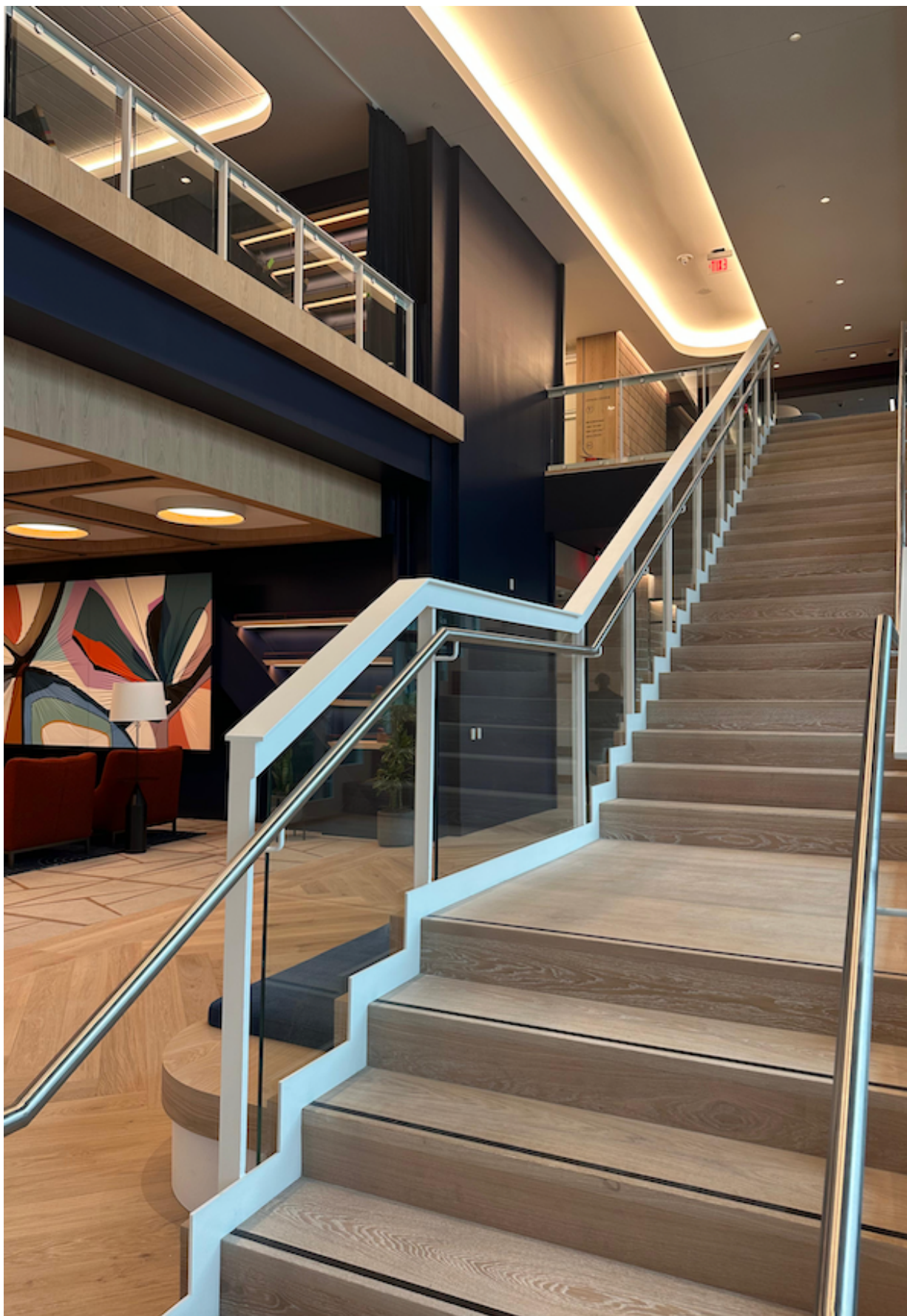
Waterfall steps with exposed ends and Wenge inlays.
