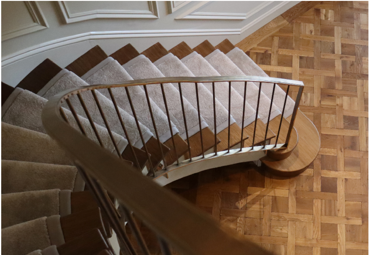
Custom bullnosed treads with a side return
